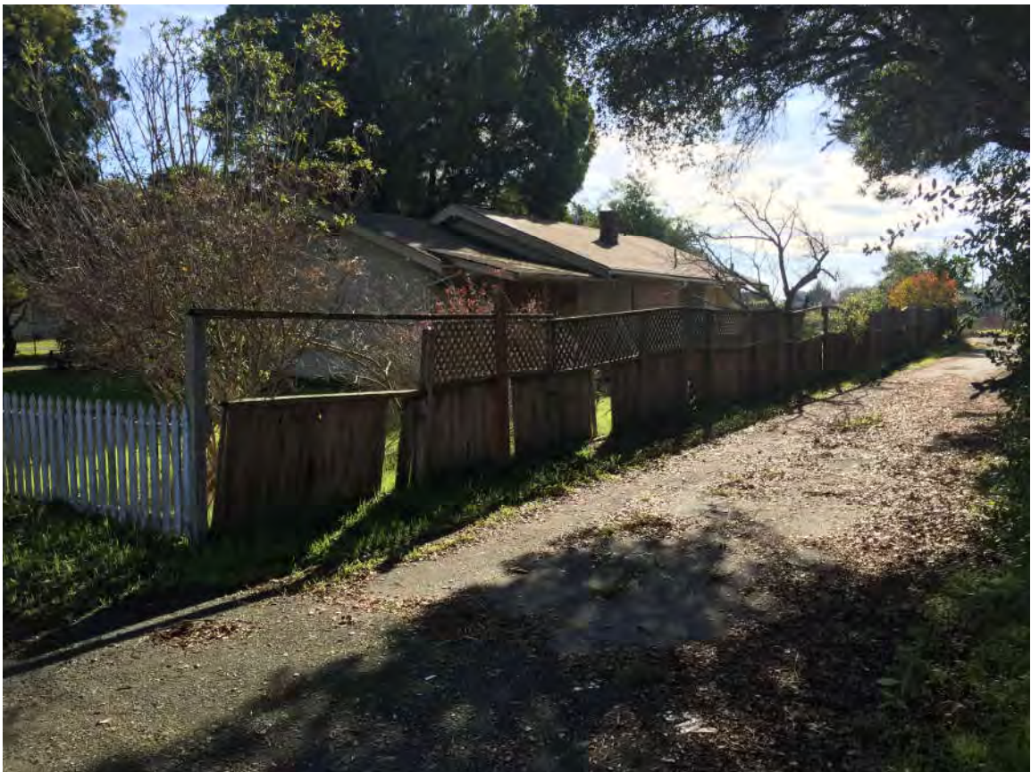
WEST DRIVEWAY AND PARKING AREA SOUTH OF HOUSE AT 1438 CAPITOLA ROAD
