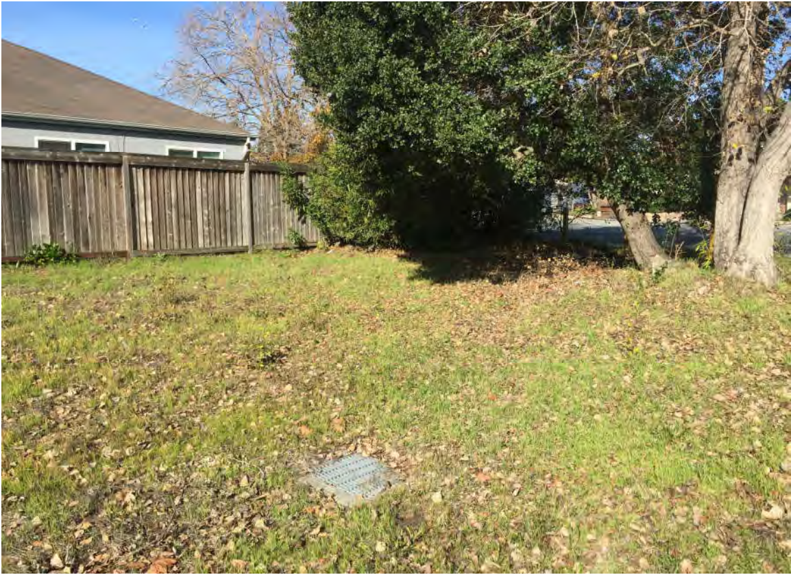
STORM DRAIN NORTHWEST CORNER OF 1412 CAPITOLA ROAD
