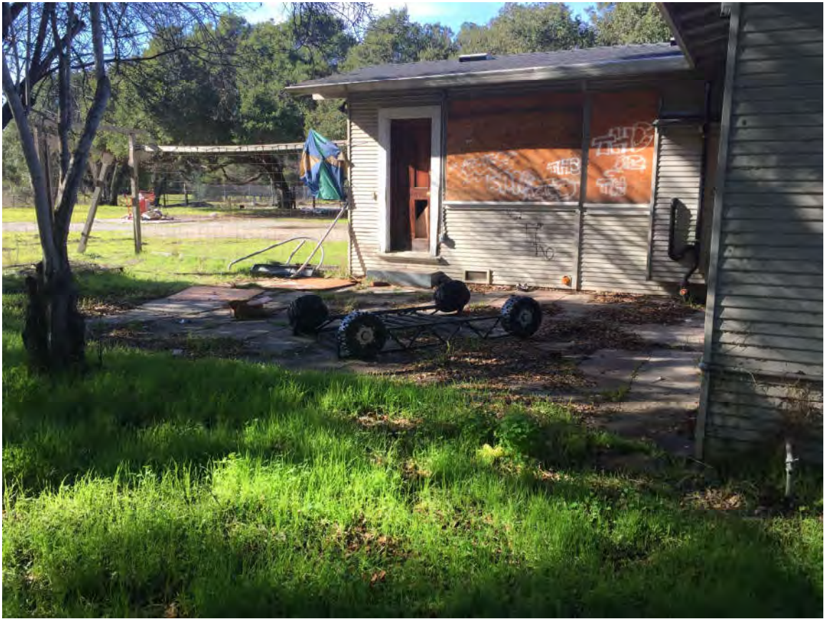
REAR OF HOUSE AT 1500 CAPITOLA ROAD
