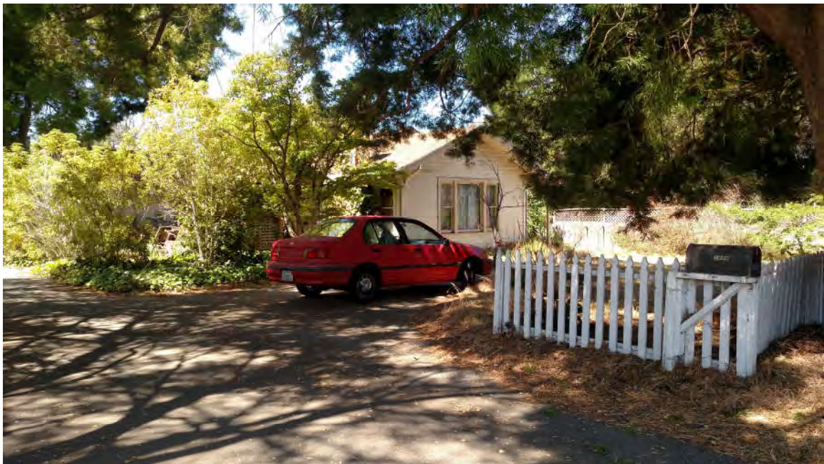
HOUSE AND EAST DRIVEWAY AT 1438 CAPITOLA ROAD VIEWING WEST-SOUTHWEST FROM CAPITOLA ROAD
